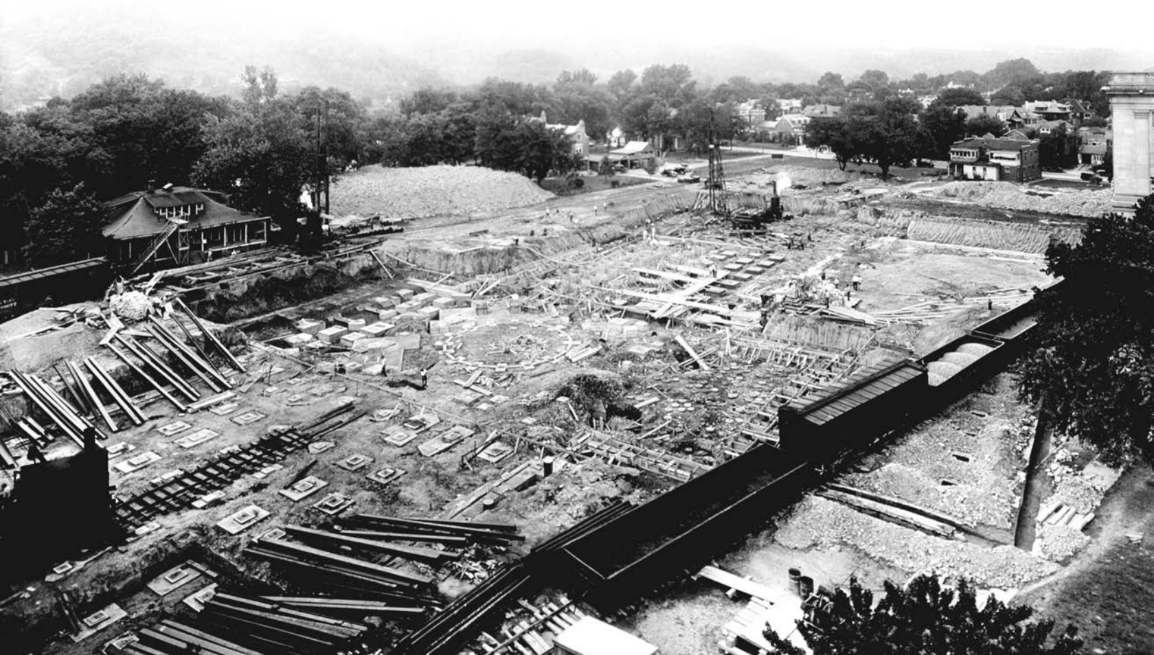
Main building excavation site, July 1930.
